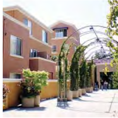
City Center Plaza, Redwood City
